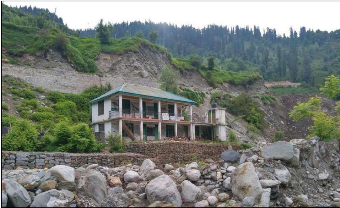
Picture 1: School building located in the hazard-prone area.
